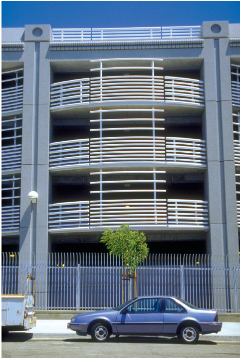
Fig. 6-3 Parking Structure adjacent to SFGHMC
