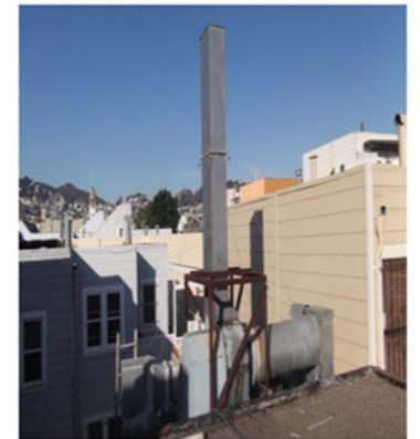
Avoid installing motors directly next to a residential window.
