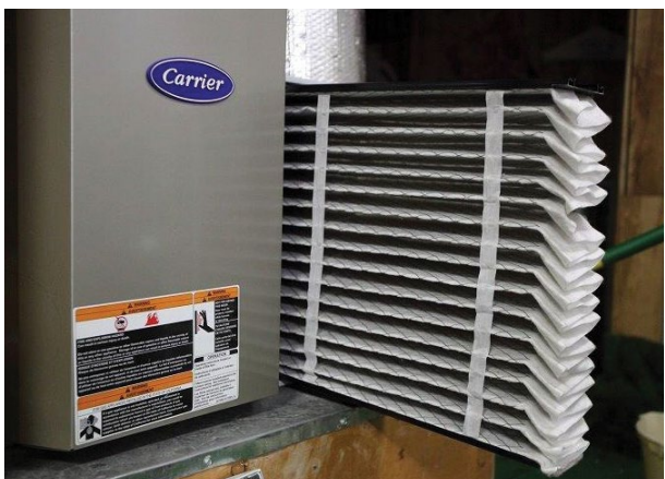
FORCED AIR FURNACE WITH HIGH EFFICIENCY FILTRATION (MERV 13 RATED)
