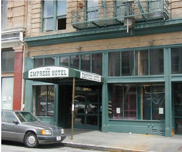
HUH's Direct Access to Housing Program provides onsite medical, psychiatric and substance abuse services for over 700 units throughout the city, including 90 units at the newly renovated Empress Hotel.
